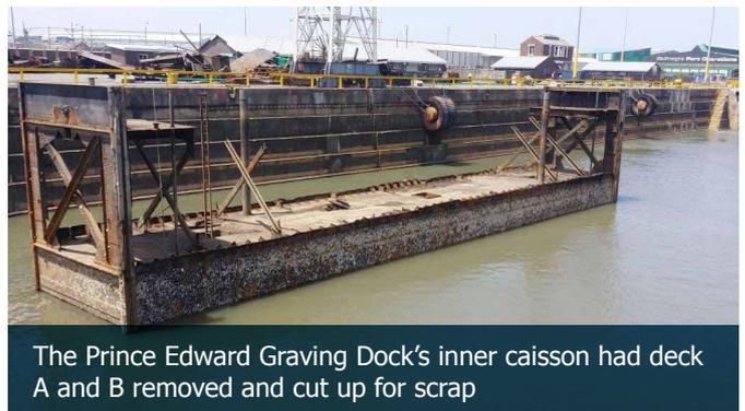
The Prince Edward Graving Dock's inner caisson had deck A and B removed and cut up for scrap
