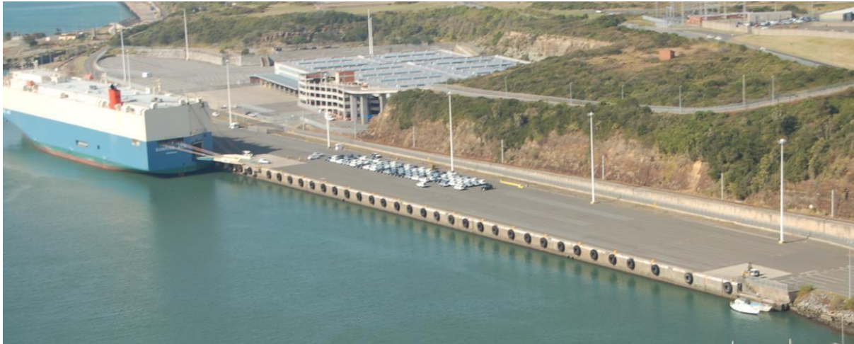
Figure 2: West Quay (Car Terminal) - Aerial Photograph captured by TNPA Corporate Affairs
