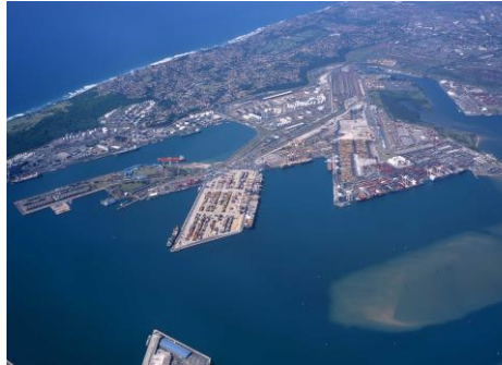
Current Pier 1 and DCT
