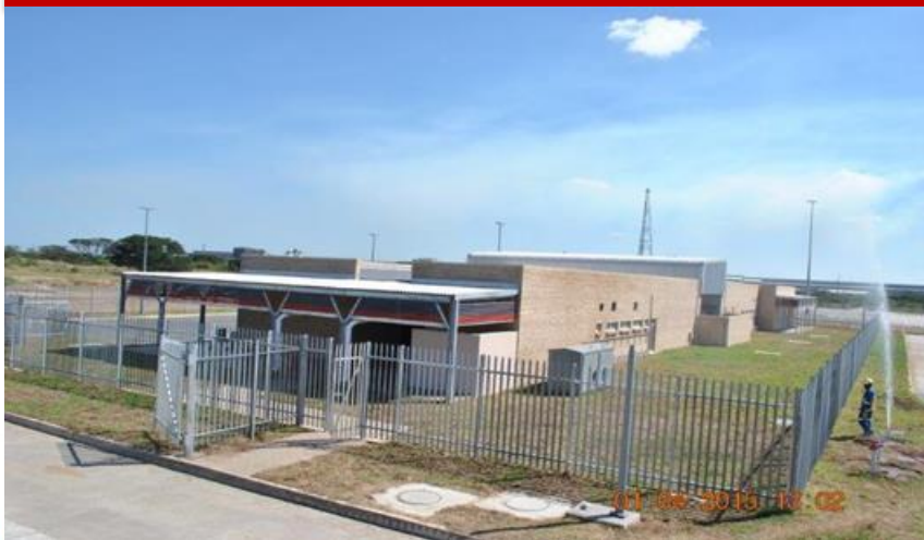
REAR ENTRANCE TO GOVERNMENT HOUSE
