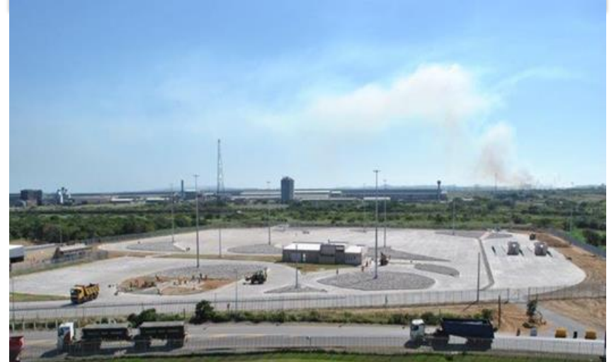
OVERVIEW OF FACILITY
