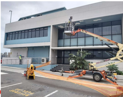
Ocean Terminal Building Repainting
