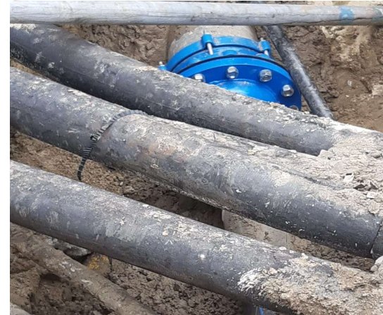
Maintenance to burst potable water pipe
