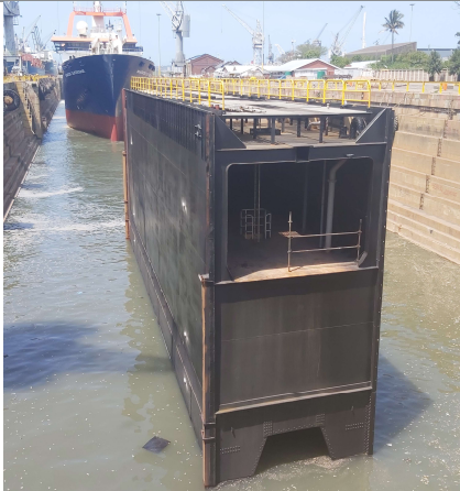
Fabrication of Dry Dock Inner Caisson
