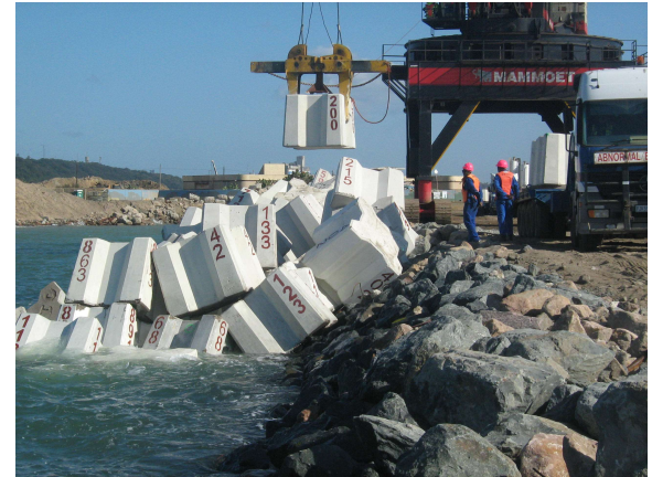
DHEW – Construction of New North Breakwater
