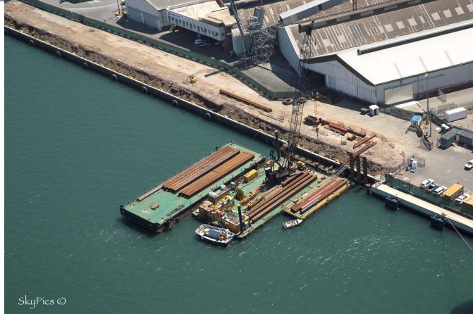
Reconstruction of Maydon Wharf Berths
